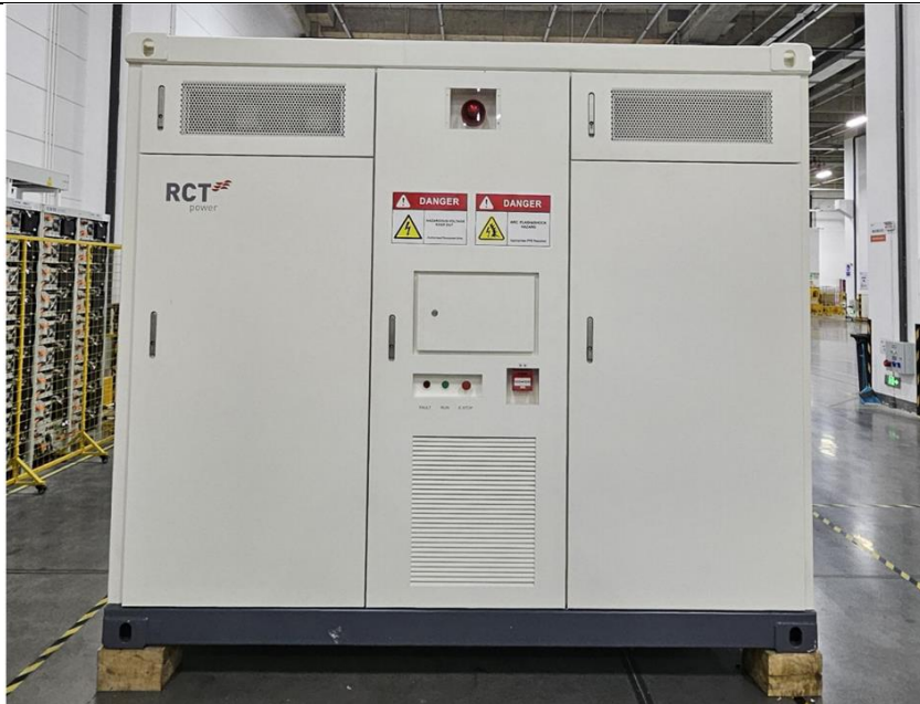
Photo 1-Overall view of CESS932-500-01D
