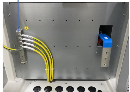
Grounding Bus Bar
