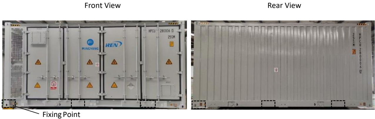
Figure 5-1 ESS container fixing points
