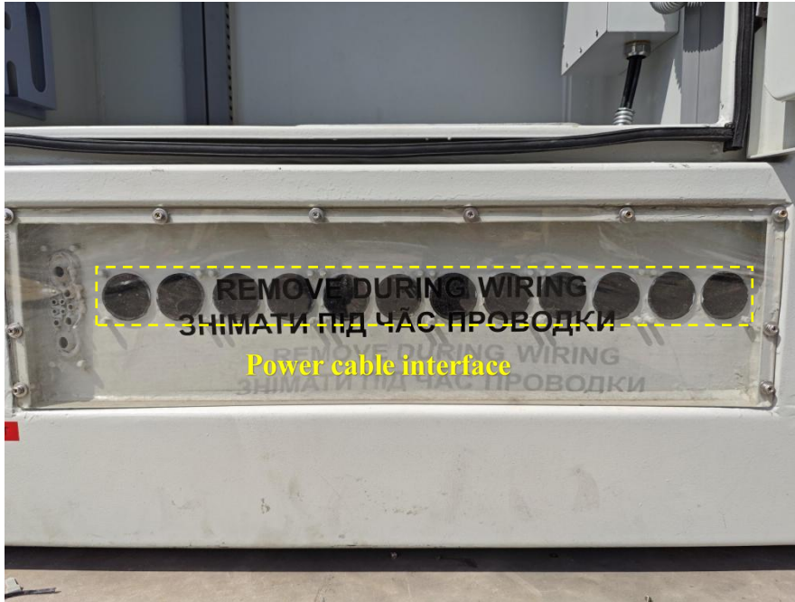
Figure 5-7 Schematic diagram of power cable interface
